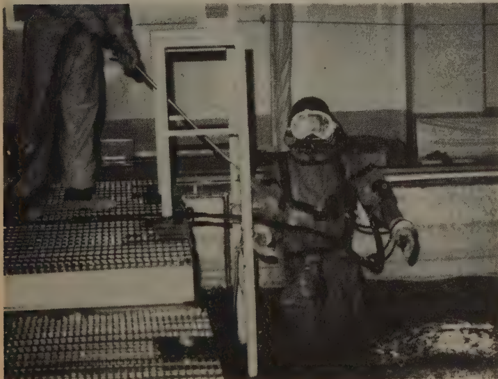
A diver being hosed off as he exits the Rancho Seco storage pool. His job was to dismantle the empty spent fuel racks prior to their removal. The spent fuel rods stored in the pool give off both radiation and heat, and his exposure time was limited by both factors.
